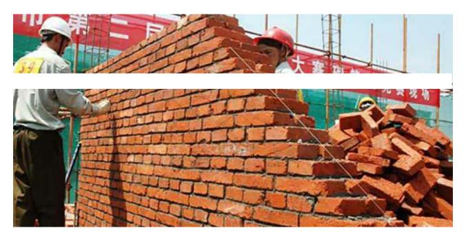
(4) The deviation of the axes of brick masonry should not be greater than 10mm, and when the building height >10m, it's 20mm.
