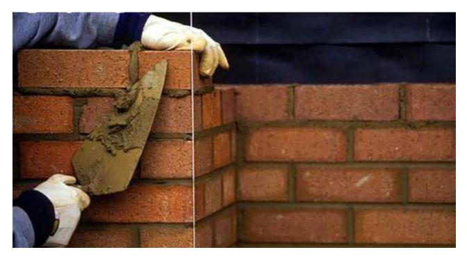
(1) The mortar plumpness of horizontal grey joints shall not be less than 80%. The bond area between brick bottom and mortar shall be checked by Baige net, and no less than 5 spot checks shall be made in each inspection batch.
